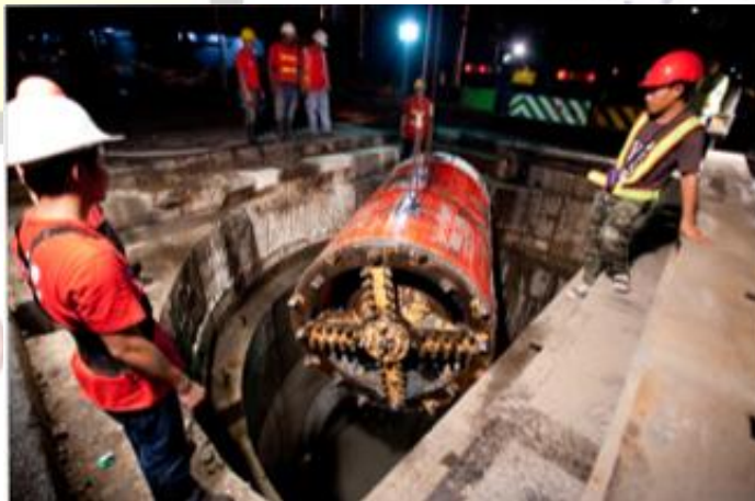
FIGURE 6.- MTBM Installation Process
